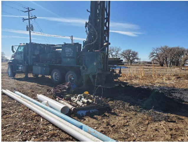
Well Inspection Report Receipt No. 10003925 page 3 of 4
